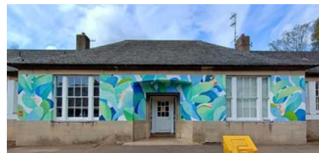
The Jordanburn entrance, after
